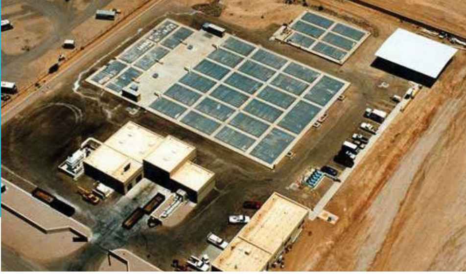
The 2.4 MGD Pima Utility Wastewater Treatment Plant meets Title 22 effluent quality standards.
