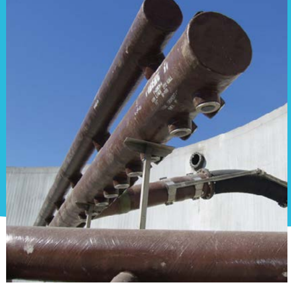
Draw tube with solids excluding plug valves.
