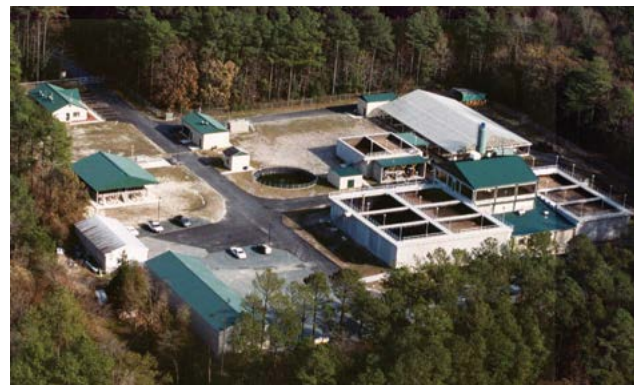
Fruitland, Maryland Wastewater Treatment Plant
