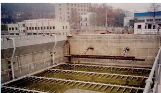
OMNIFLO® SBR with Coarse Bubble Diffusers
