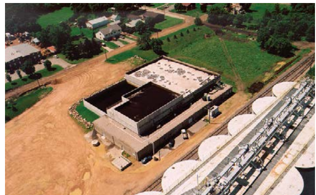
OMNIFLO® SBR installed at Rahr Malting
