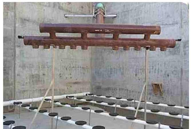
OMNIFLO® SBR with Fine Bubble Diffusers
