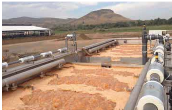
ADI Systems' packaged membrane tank is shipped with all internals and membrane cassettes pre-installed, resulting in a short turnaround from delivery to generating solids-free effluent. Photos by Evoqua/ADI
