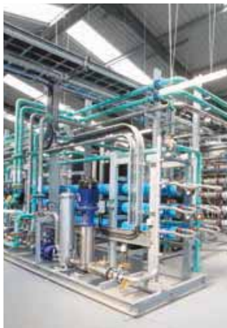
Reverse osmosis filtration at the Cucina Sano water recovery facility Photo by Aquabio
