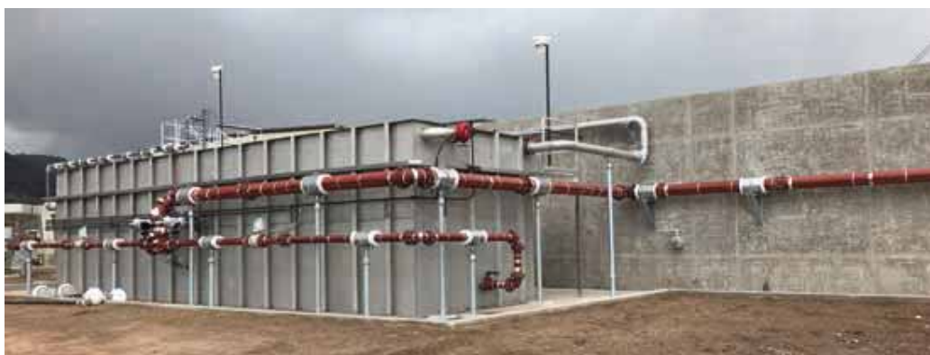
The prefabricated membrane tank is compact and provides a plug-and-play approach to water recovery. Photo by Evoqua/ADI
