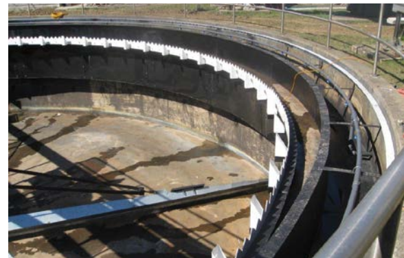
Conversion of center effluent arrangement to peripheral influent/effluent channel design
